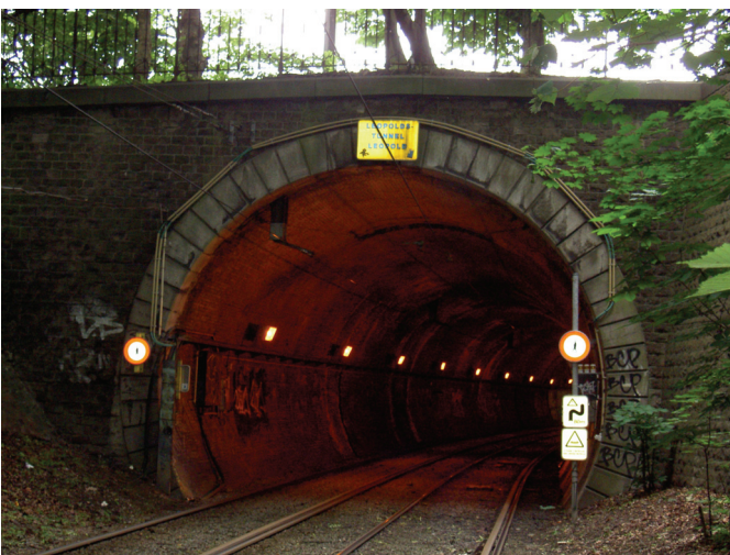
Leopold II tunnel
